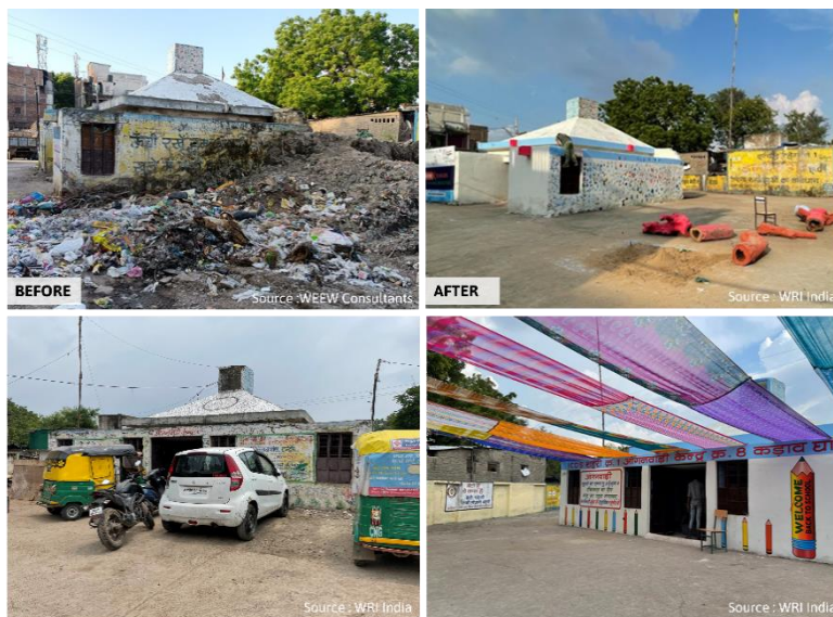
Figure 16: Reclamation of public space at anganwadi in Indore Image Source: WEEW Consultants, WRI India
