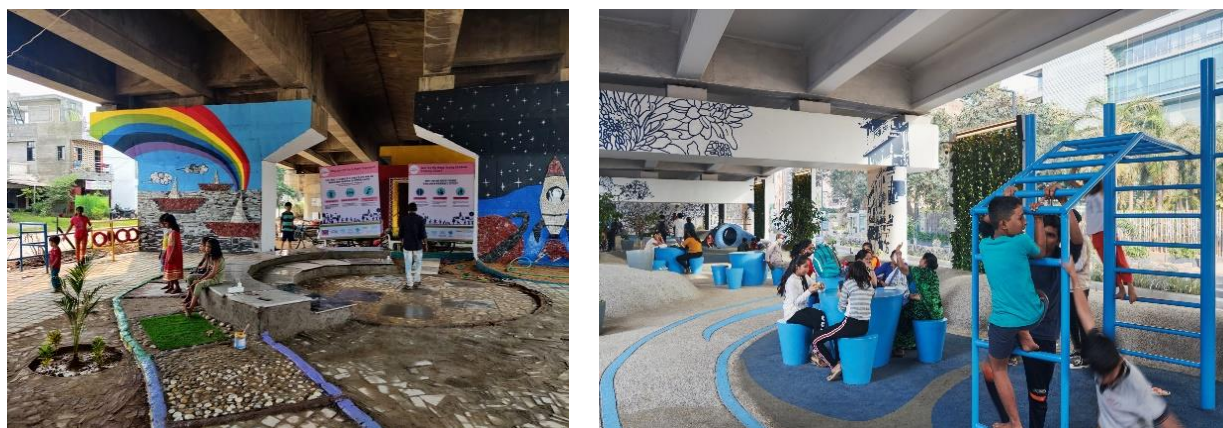
Figure 13: Transformation of neglected spaces such flyover under spaces in Vadodara and Mumbai
